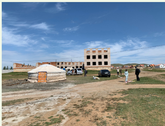
Future site for one of family health centers. One of the project sites where ground source heat pumps will be introduced to new family health centers. Test drilling and thermal response tests were conducted in August 2019 at the location. (Photo credit: ADB)
