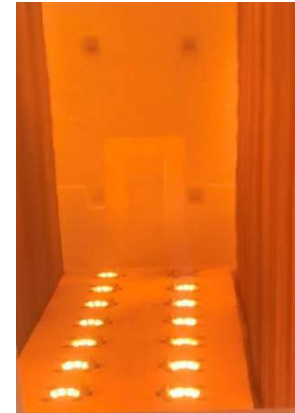
Current generation burner firing 80-85 vol. % Hydrogen
