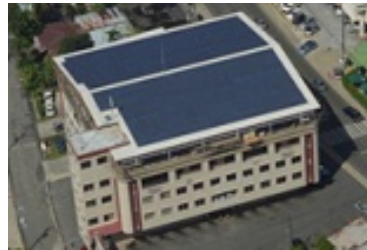
Installing solar PV system, PCKK, Palau Maldives
